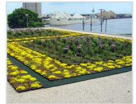
Green roof - after.
