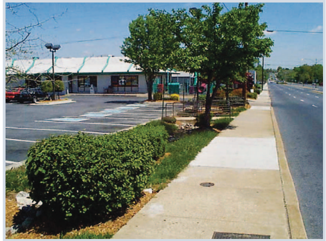
Biofiltration installation.
