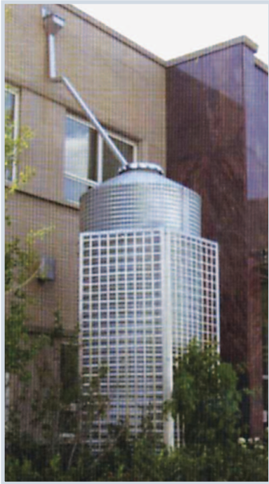
Roof water cistern.
