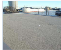
Green roof - before.
